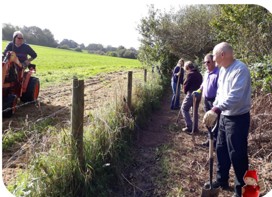
Merriott Footpath Group volunteers working on footpath surface improvements
